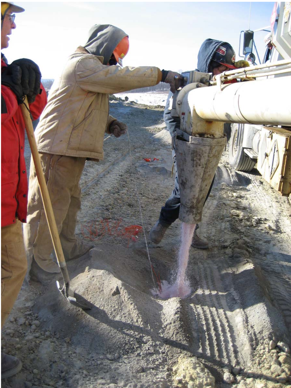
Figure 12 – Loading a Blast Hole with ANFO
