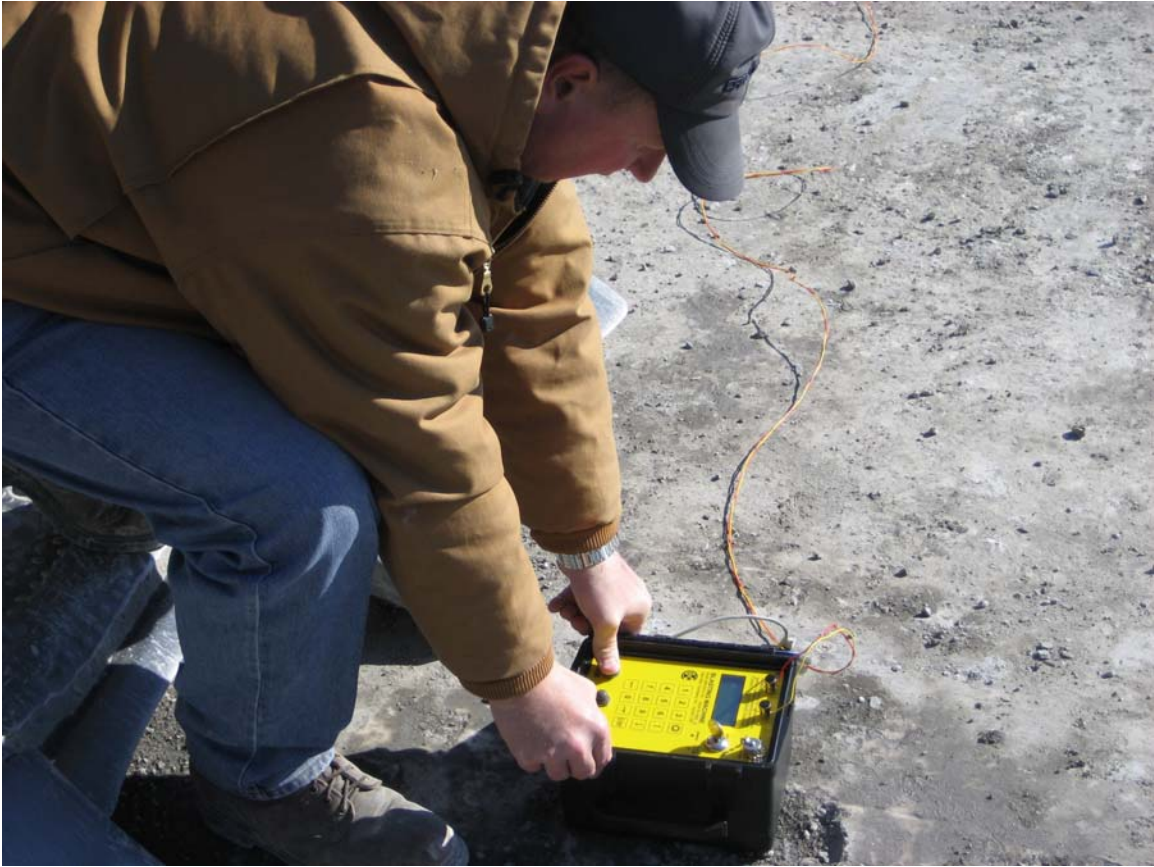
Figure 14 – Arming and Firing the Dan-Mar Digital Blasting Machine
