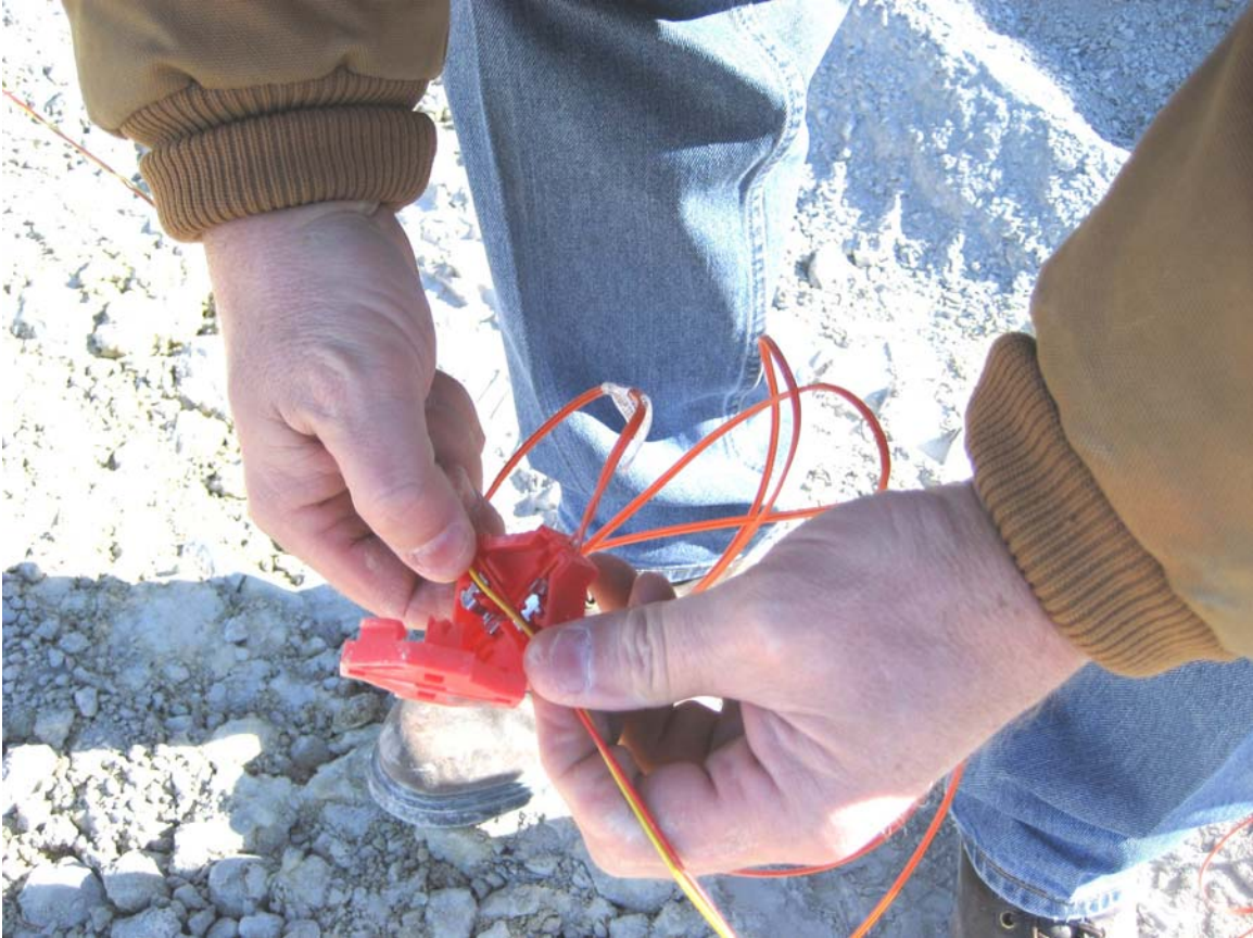
Figure 13 – Connecting an E*Star Electronic Detonator to the Buss Line
