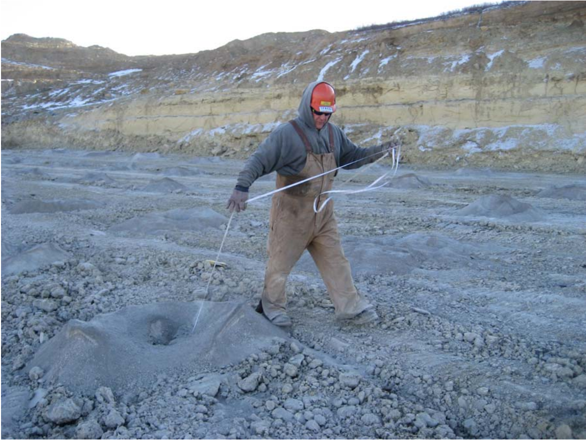
Figure 10 – Check on Depth of Blast Hole
